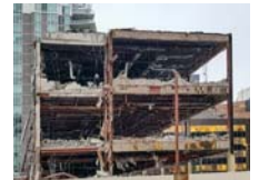
Sam Livingston building is under demolition
