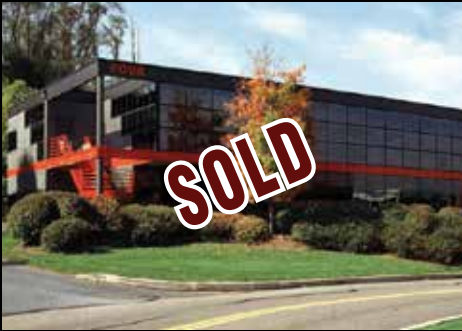
4 Lemoyne Drive, Lemoyne, PA 1,450 SF to 4,094 SF available for lease. Terrific floor to ceiling windows.
