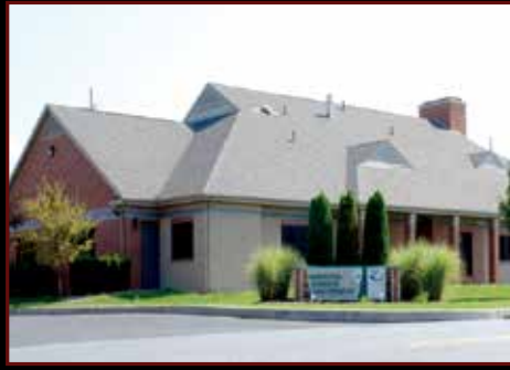
2704 Commerce Drive, Harrisburg, PA 1,000 to 10,000 SF available. High end finishes throughout. Ample on site parking.
