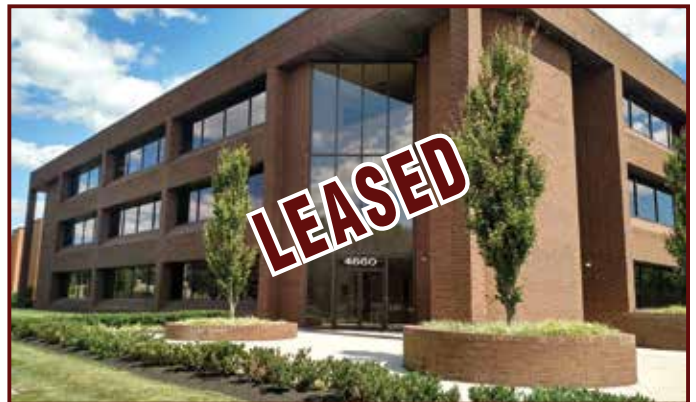
4660 Trindle Road, Camp Hill, PA
