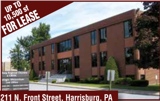
3211 N. Front Street, Harrisburg, PA
